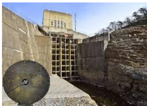
The gage, gate & creek.
