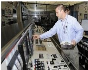
Power plant control rooms
